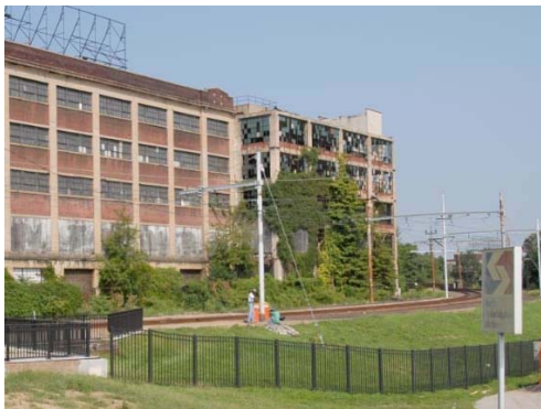
Under-utilized site adjacent to North Philadelphia Amtrak / SEPTA stations
